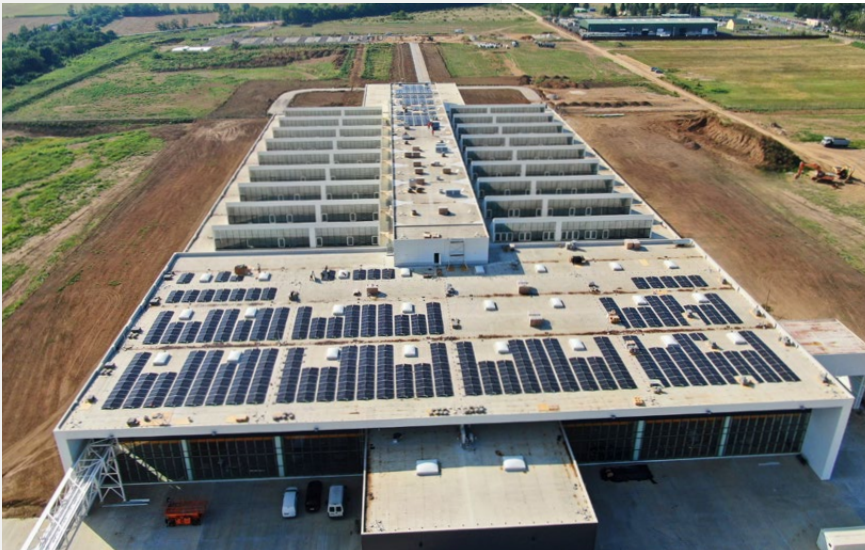
The new production site in Szombathely in Western Hungary is the Schaeffler Group's first plant dedicated entirely to e-mobility.
